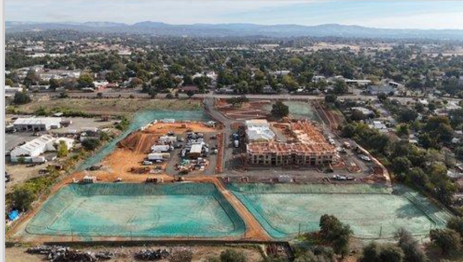
Lincoln St. Phase 1, Sunseri Construction
