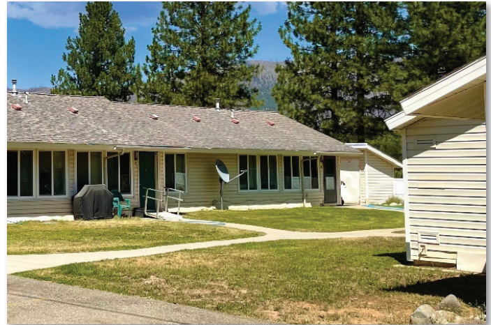
One-story courtyard-style multi-family construction, similar to these existing units in Greenville are typically more cost-effective than multi-level construction and provide access to outdoor space for families with children.
